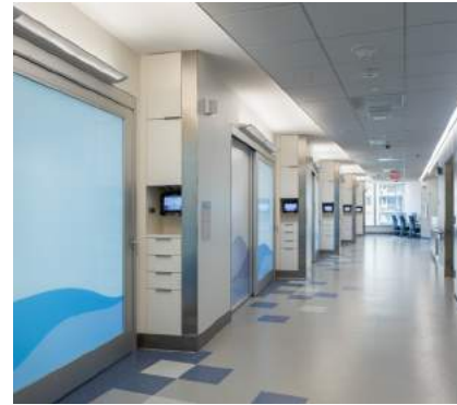
Recycled content included with acoustic ceiling tiles Regional material and Greenguard resilient flooring
