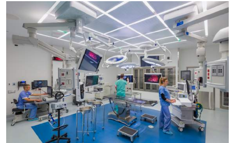
Operating Room includes full lighting and thermal comfort temperature controls. Low emitting paints and flooring. Occupancy sensors to allow the air change rates in the space to be reduced when the space is not in use.
