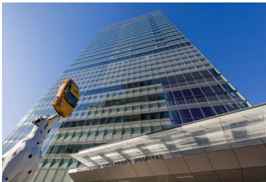
Hassenfeld Children's Hospital - Jeff Goldberg/Esto
